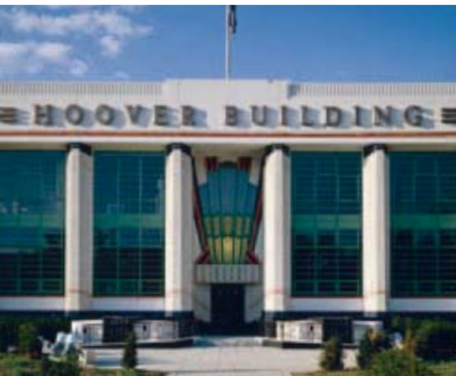
Office and factory for the Hoover company This 1933 landmark London building by architects Wallis, Gilbert, and Partners has an American-style glazed Art Deco façade and a striking, brightly coloured, Egyptian-style faience over its entrance.
