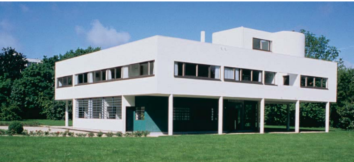
Villa Savoye, Poissy-sur-Seine This is an early and classic example of Modern architecture. Typical of what became known as the International Style are the strip windows, flat roof and deck, and rectilinear lines of the design. Designed by Le Corbusier and Pierre Jeanneret. 1929–30.
