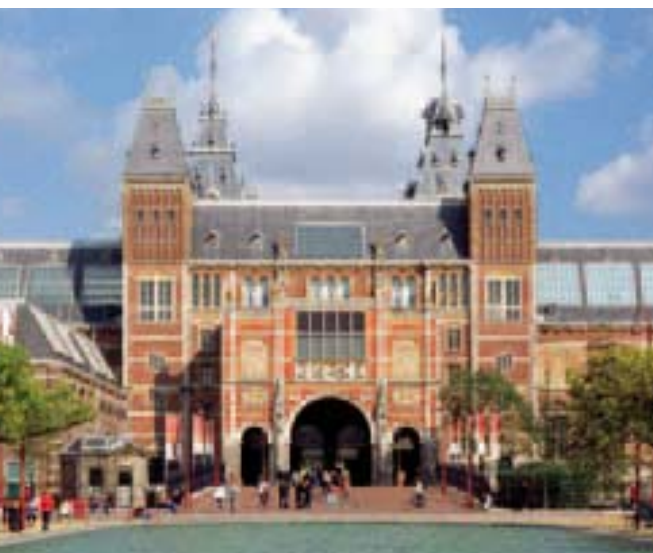
West facade of the Rijksmuseum, Amsterdam Designed by Pierre Cuyper to house the national art collection, the building opened to the public on 13 July 1885. It is a combination of Romanesque, Gothic, and Dutch Renaissance styles.
