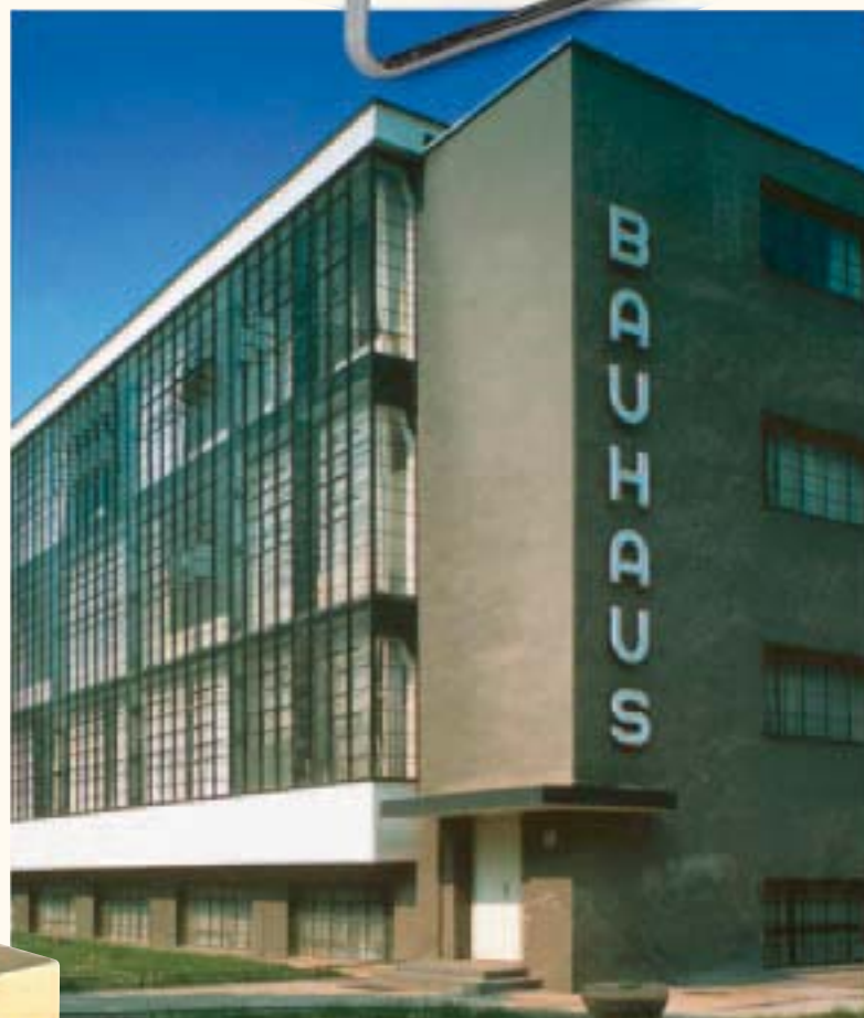
Gropius's and Meyer's industrial-looking masterpiece for the Bauhaus School The dominant feature of this building was its steel-and-glass façade. It was testament to the Bauhaus belief that form should follow function.
