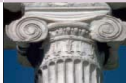
Ionic capital at the top of a column, part of the Parthenon, Athens.
