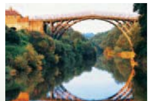
The world's first iron bridge This bridge was erected over the River Severn at Coalbrookdale in Shropshire, England in 1779.
